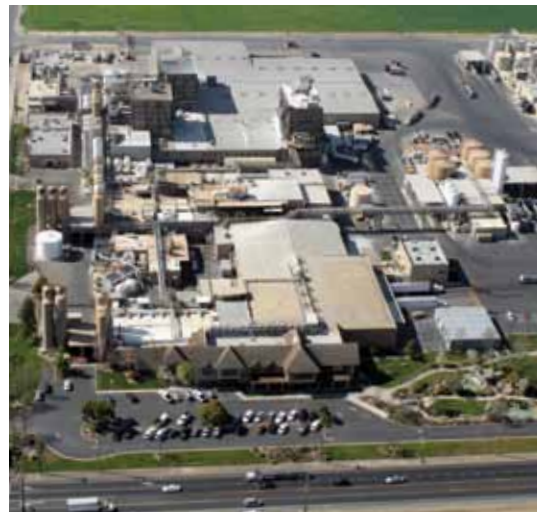
Hilmar, CA, facility 2011
